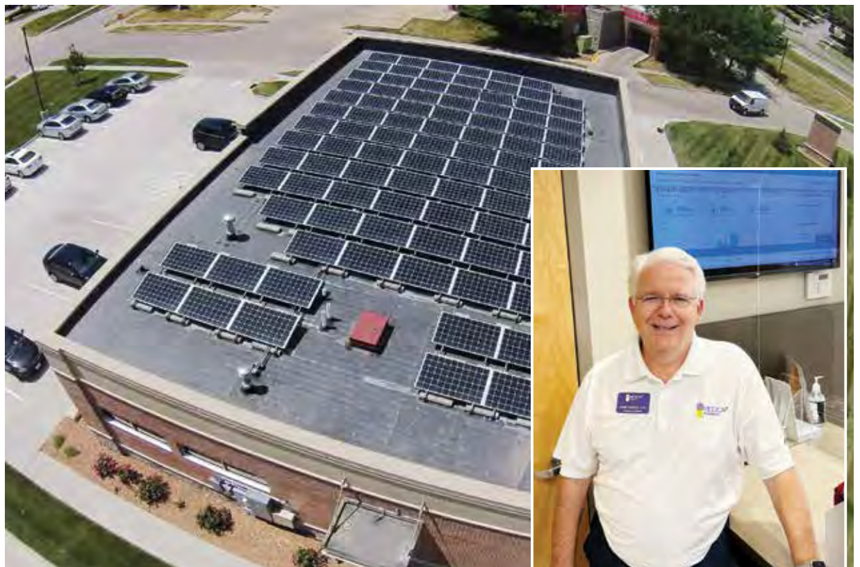
Medicap Pharmacy in Urbandale has 90 total solar panels on its roof. Photo courtesy of John Forbes
