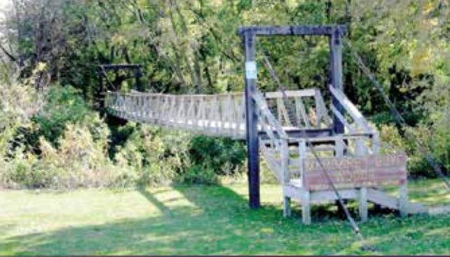
Guye Woods suspension bridge
